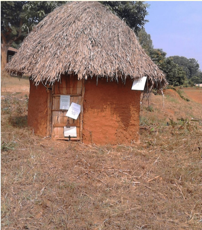
Figure 1: Constructed Storage House (SH).
