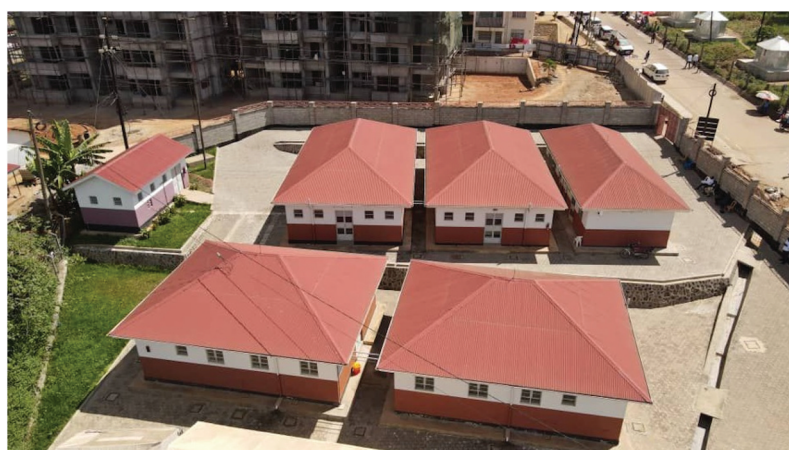
Figure 3. Photo of the isolation unit built at Mbarara Regional Referral Hospital through the support of First Mile.
